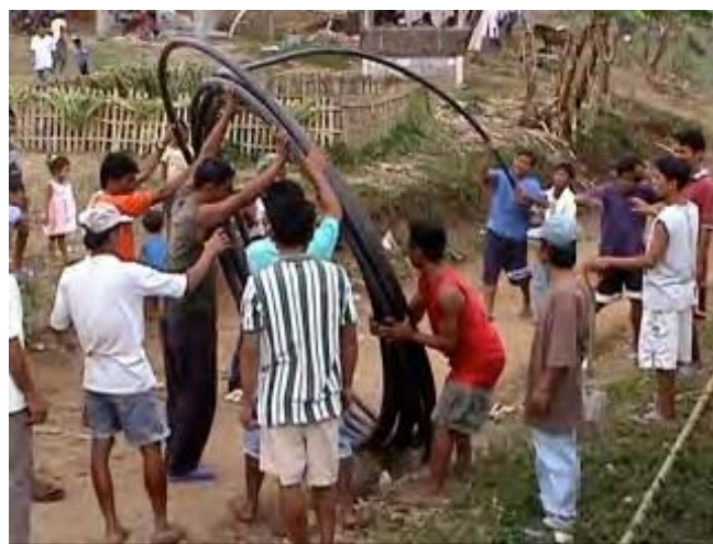
A nearby UU community laying a pipe in Nagbinlod
