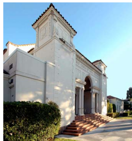
The prospective new building on Oak Grove, Burlingame
